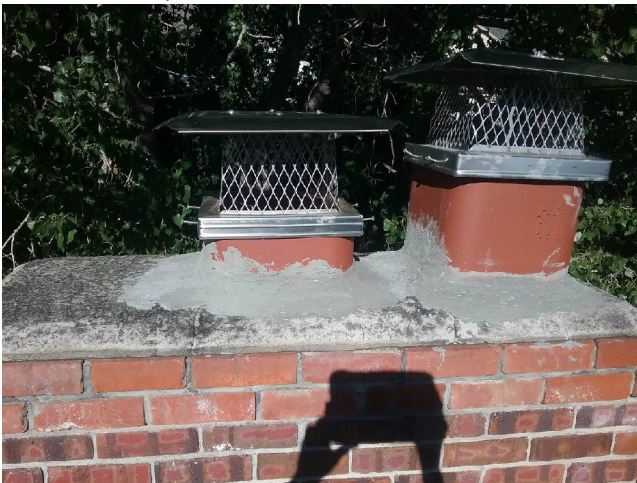
Chimney Flashing: Galvanized
