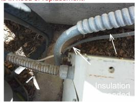
18. 2029 AC System Refrigerant Lines: Repair - 1. The exterior AC unit's refrigerant line insulation is in need of replacement.
