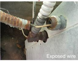
20. 2031 AC System Refrigerant Lines: Repair needed - 1. The exterior AC unit's refrigerant line insulation is in need of replacement.
