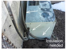
15. 2021 AC System Refrigerant Lines: Repair needed - 1. The exterior AC unit's refrigerant line insulation, unit 2021 is in need of replacement.
