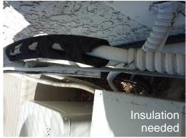
17. 2027 AC System Refrigerant Lines: Repair needed - 1. The exterior AC unit's refrigerant line insulation, unit 2027 is in need of replacement.
