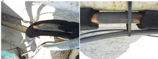
16. 2025 AC System Refrigerant Lines: Repair needed - 1. The exterior AC unit's refrigerant line insulation, unit 2025 is in need of replacement.
