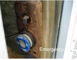
Gas Shut Off: Yes See picture. You can turn the handle a quarter turn to shut off the valve. When the handle is in line with the pipe it is on and when it is perpendicular with the pipe it is off.
