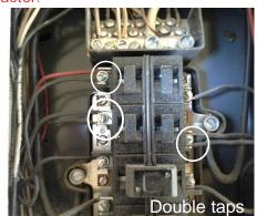
24. 2025 Electric Panel Manufacturer: Push-O-Matic - 1. Two wires are connected to a breaker designed for only one wire. This is known as a double-tap and is a defective condition which should be corrected by a qualified electrical contractor.
