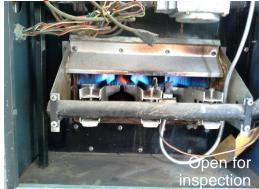
8. 2027 Heating System Heating System Operation: Adequate - 1. Due to the age of the furnace we recommend a licensed HVAC tech inspect the furnace and heat exchanger.
