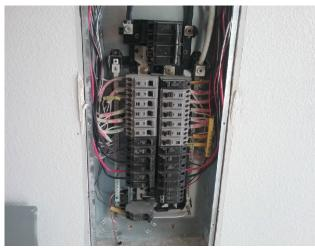
Maximum Capacity: 200 Amps Main Breaker Size: 200 Amps -Note: The main breaker is located in the main electrical panel.
