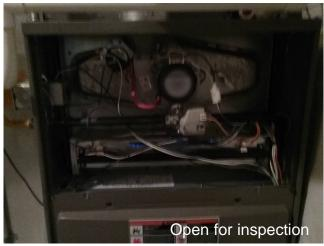
Manufacturer: Lennox Type: Forced air Capacity: 132,000 BTUHR Area Served: Whole house Manufaction Year: 2015 Permit Pulled: Yes -Permits are required to be pulled for the installation of any furnace.
